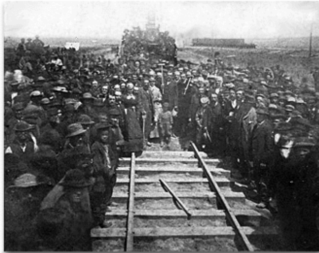
The Last Rail is Laid
